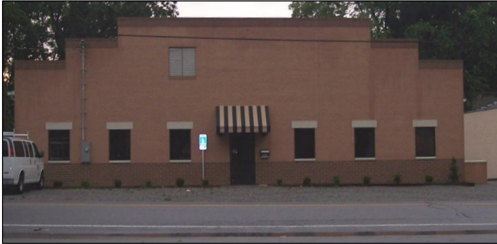
Davies Commercial Masonry
