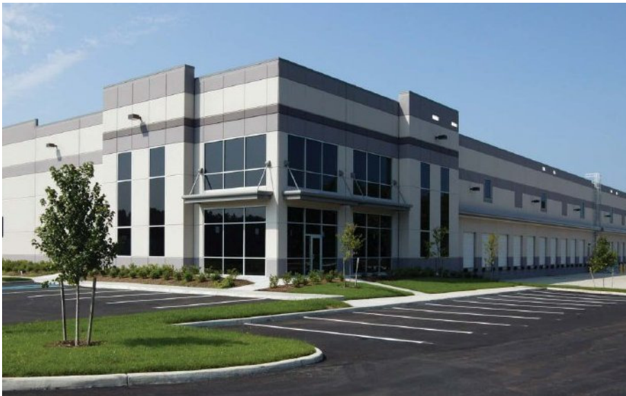
Virginia Commerce Center, 375 Kenyon Road, Suffolk, VA 23434
